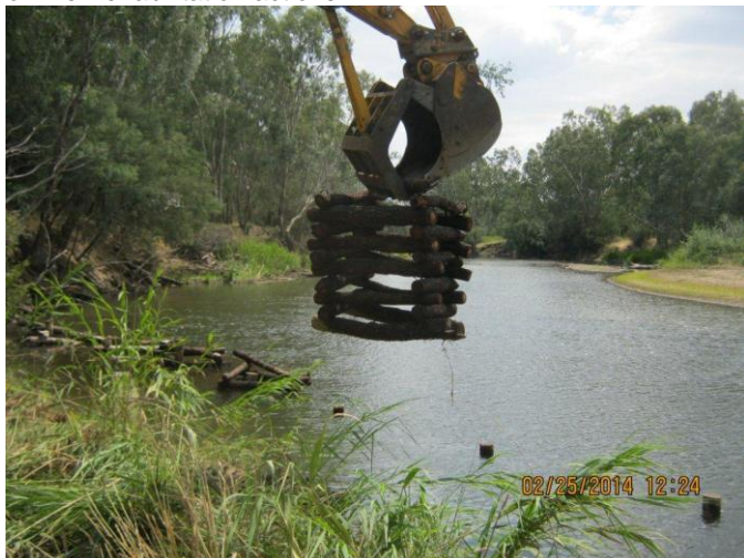
Inserting fish hotels into the Ovens River to increase native fish habitat. Photo: A. Wilson
